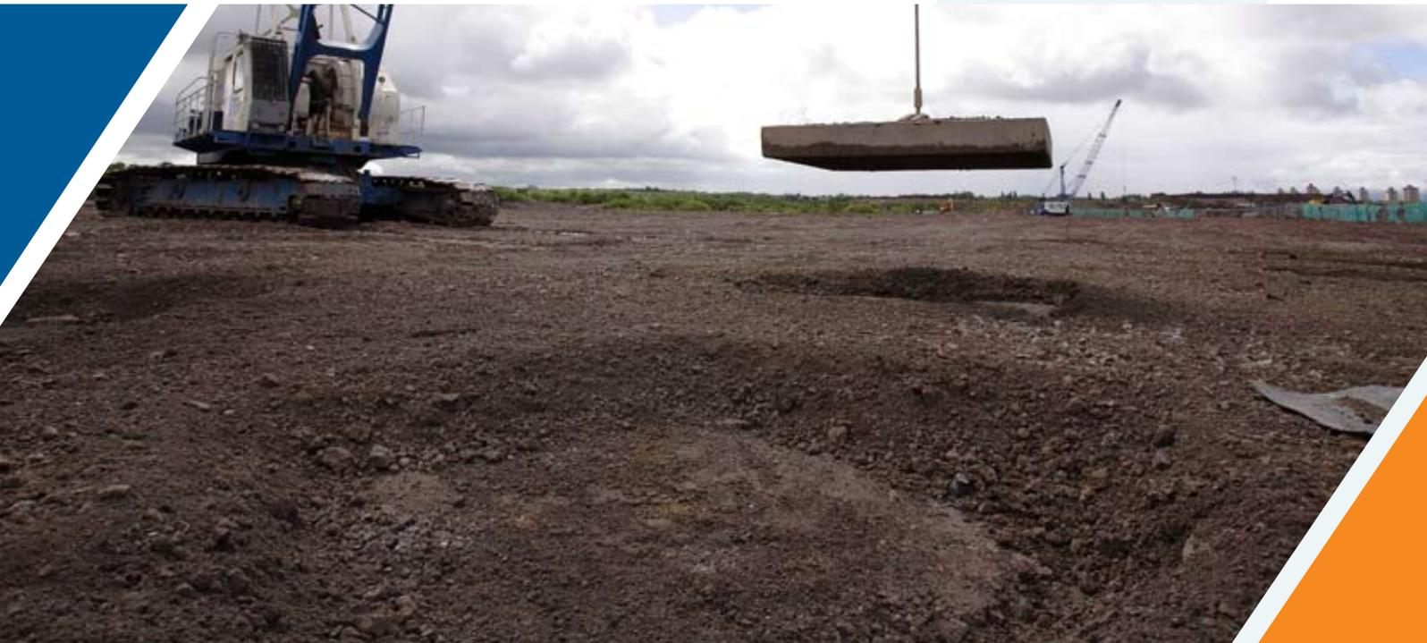
Dynamic Compaction (DC) is the use of high energy tamping to induce settlement in a wide variety of ground conditions from loose granular materials to mixed made ground, including domestic landfills.
